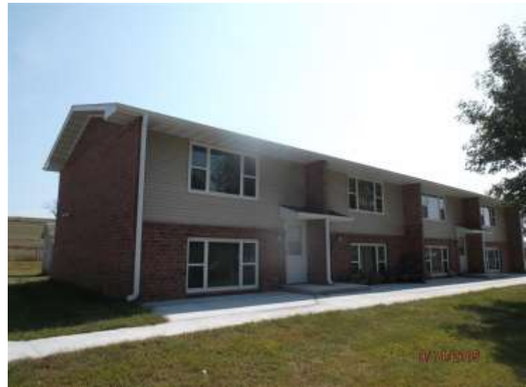
After the Renovation, 2012
